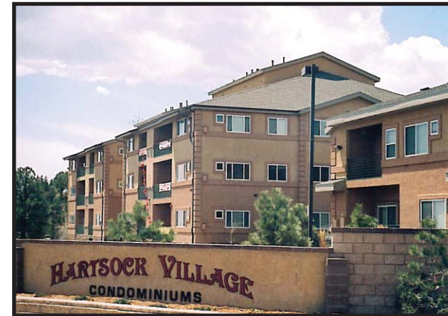
Hartsock Village Condominiums
